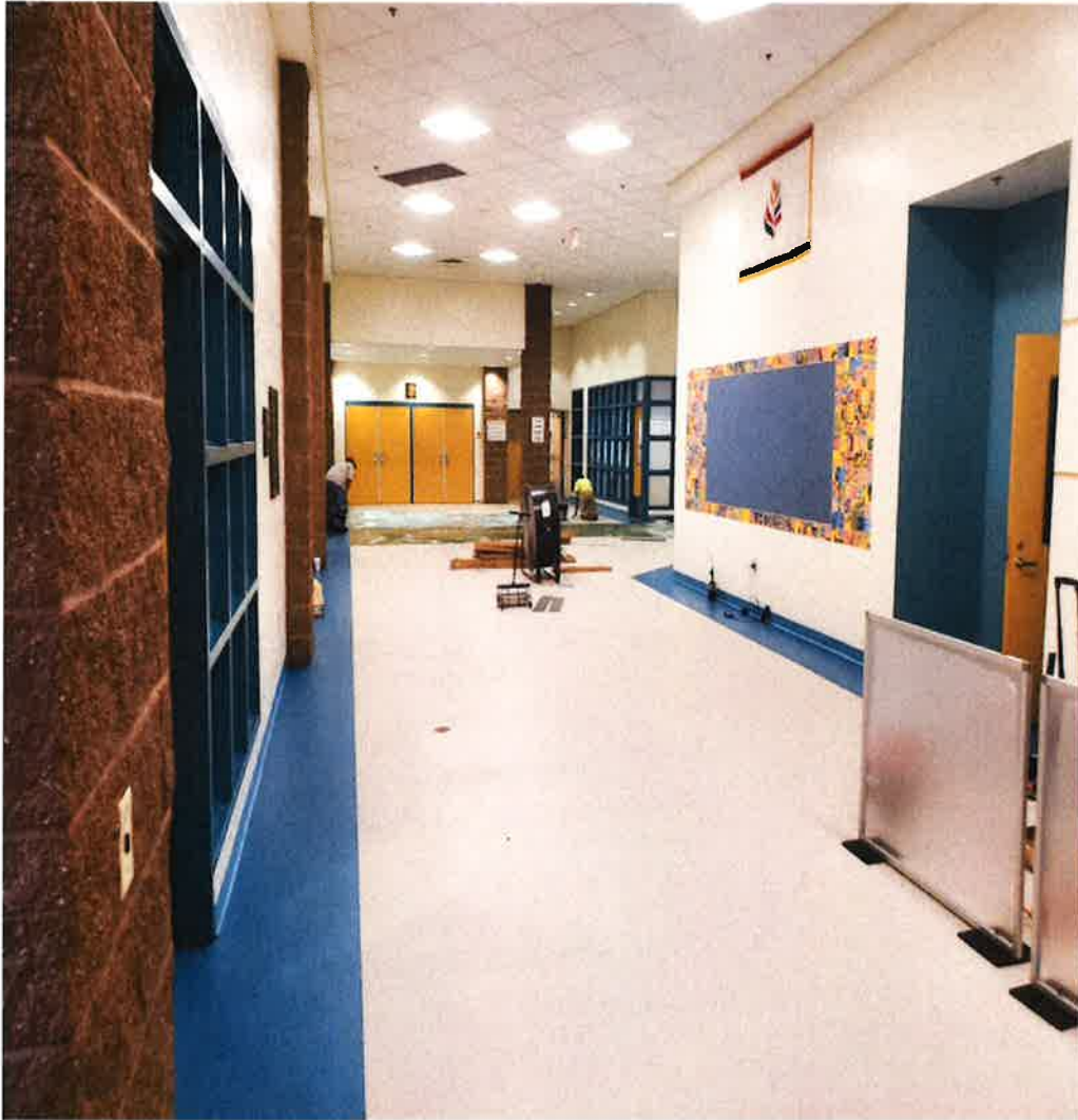
Reed Intermediate – New flooring in main lobby
