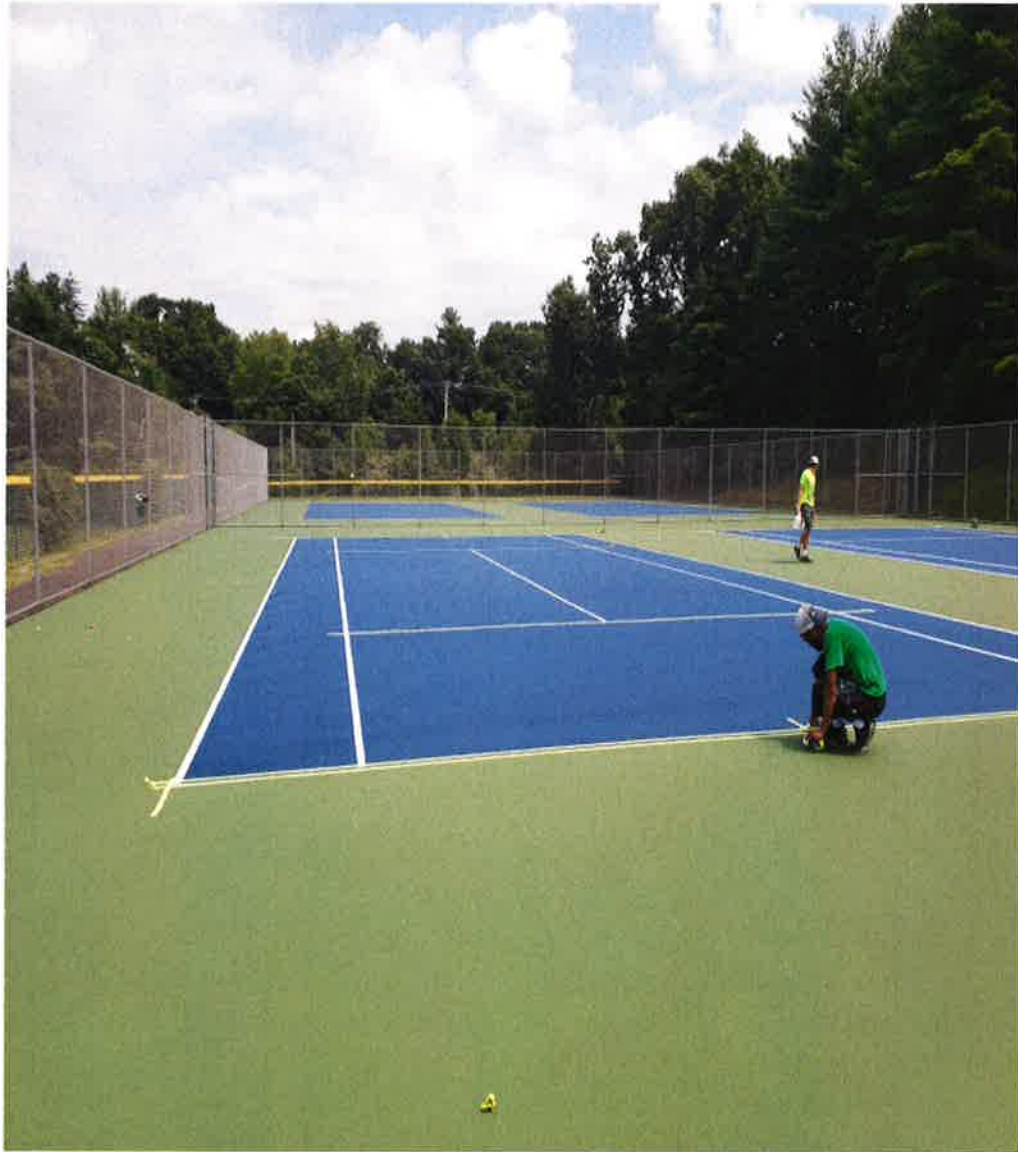
Newtown High School – Resurfaced tennis courts
