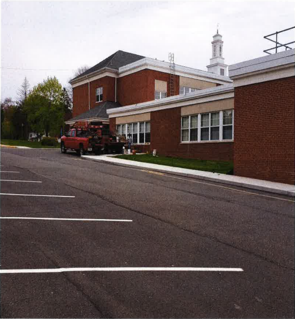
Newtown Middle School – Repointed mortar joints
